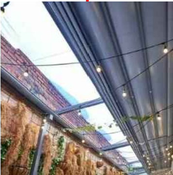
WEATHERPROOF, RETRACTABLE ACOUSTIC FABRIC ROOF TO OPEN GABLES to future detail Image indicative only Colour: Charcoal
